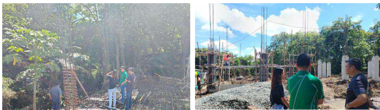
Figure 47. 4th Quarter 2025 Construction Progress
