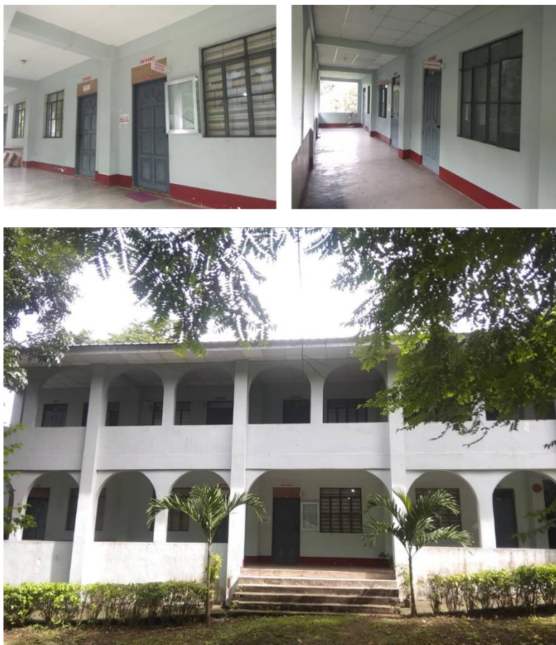
Figure 4 Current Engineering Building
